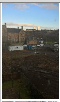
The remaining external walls of the old Springburn Public Halls which are being excavated and removed to allow the piling to start next year.
