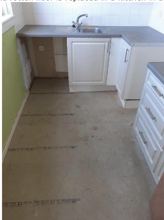
A damaged and rotten floor is replaced in a kitchen in a void property
