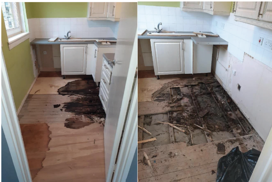
A damaged and rotten floor is replaced in a kitchen in a void property
