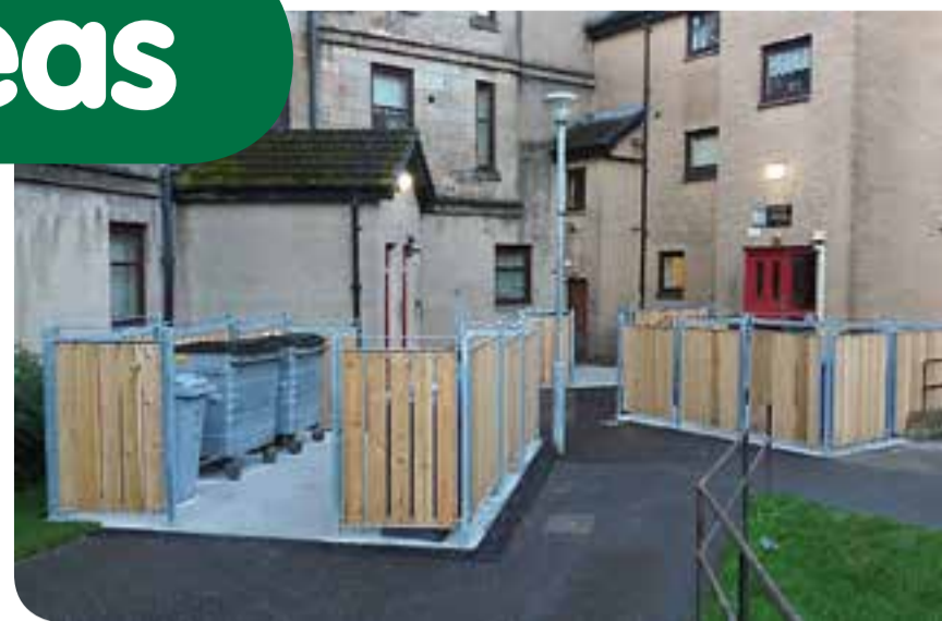
Kemp Street - After
