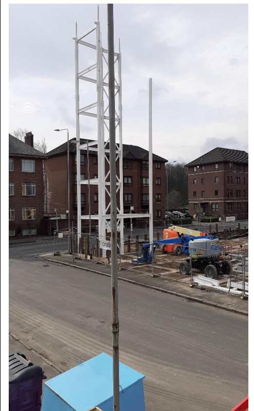
The new steel frame has started being erected.
